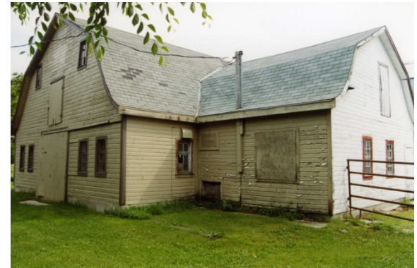
Figure 45. Ste. Anne-area barn, once used for dairy cattle and now for dances. The distinctive gambrel form used for the barn is reinforced in the section over the main doors (top) and then also in the junction of two sections (bottom) where the complexity of the form gains more prominence.
