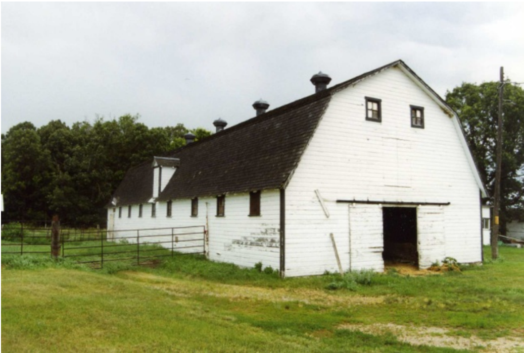
Figure 44. Notre Dame de Lourdes-area dairy barn.
