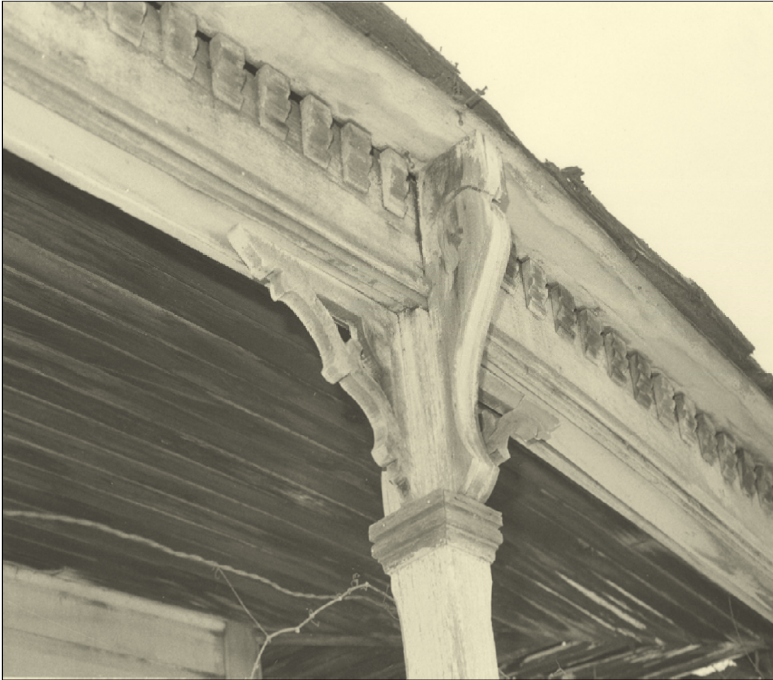
Figure 27 Roddick House. The intricate post caps on the veranda created a sense of lightness.
