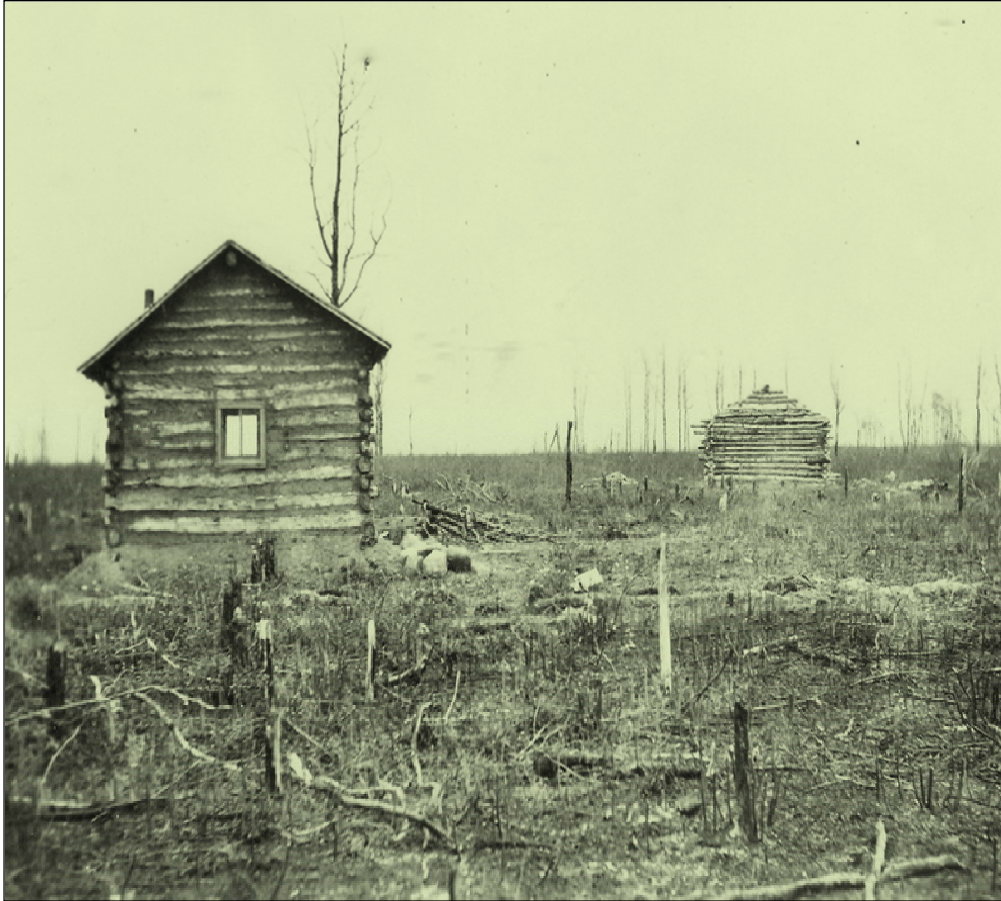
Figure 8 Reverend Roddick log cabin, SE 17-9-18W, ca. 1879. This house was probably one of the first built in the planning district, and this image suggests the rough pioneer experience. (Murray McPherson.)
